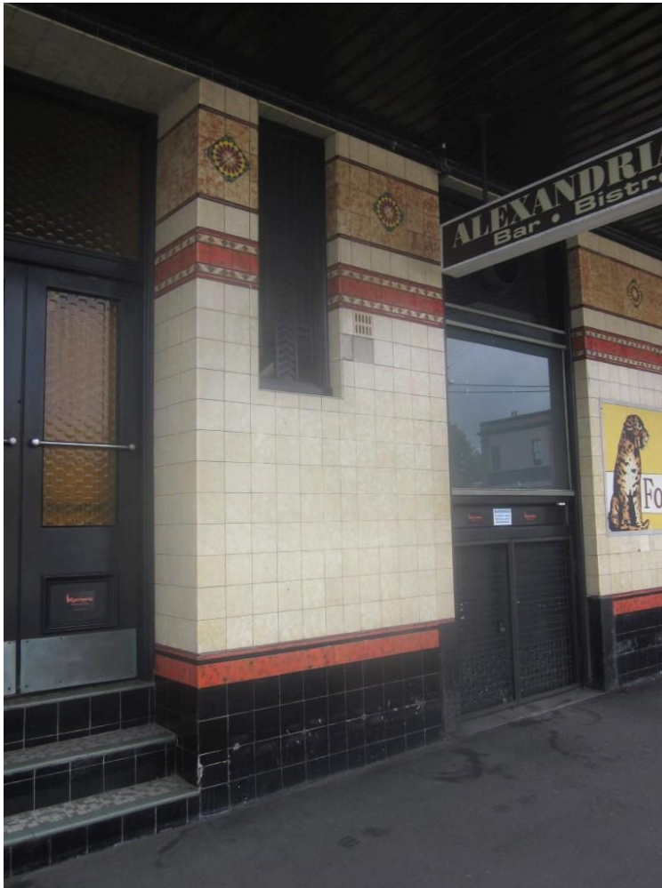
Figure 19 Intact wall tiles and joinery on the Henderson Road facade.
