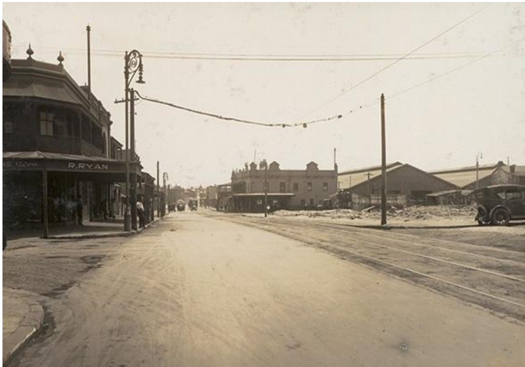
Figure 6 Demolition along the northern side of Henderson Road between Wyndham and Garden Streets, 23 November 1927. The Alexandria Hotel can be seen in the centre of the photograph and is yet to be demolished.
