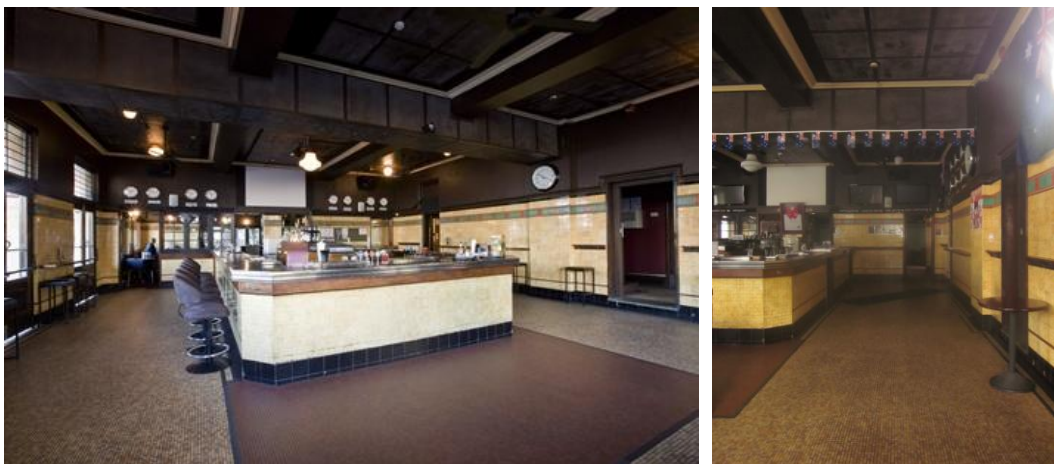
Figure 20 The public bar. Original fabric that remains in place includes wall and floor tiles, a part of the bar, and glazed joinery that formerly separated the bar from the bottle sales area. The ceiling has undergone some modification, although early fabric may be concealed behind later linings. The original extent of the bar area is indicated by the dark-toned floor tiles.
