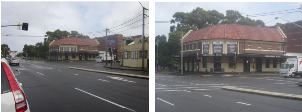
Figure 17 The Alexandria Hotel viewed from the east on Henderson Road.
