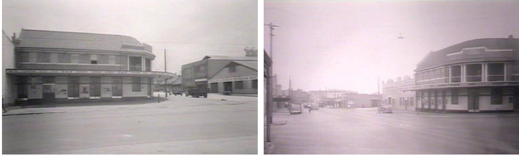
Figure 14 Views of the Alexandria Hotel in the context of Henderson Road and Garden Street, December 1936 and August 1939
