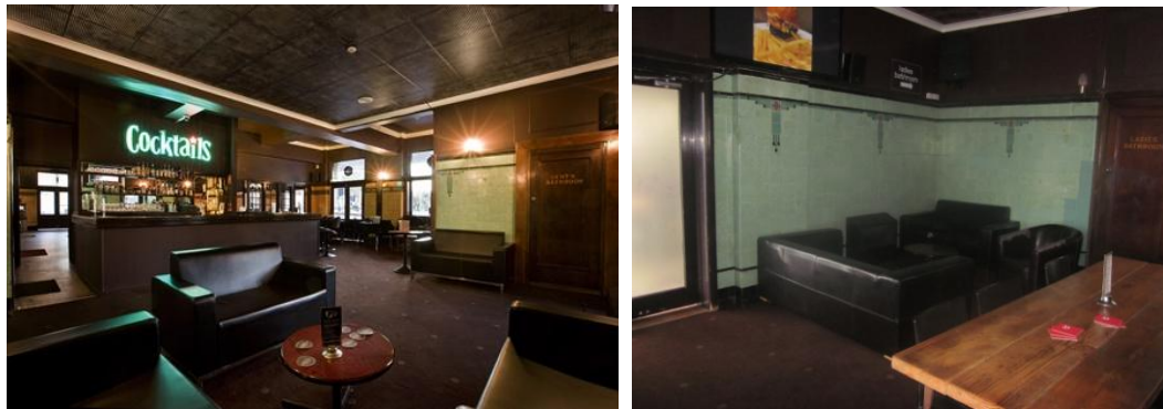
Figure 21 Former saloon bar. The bar area is not original, and the space has been opened up to the public bar. Wall tiles are original.
